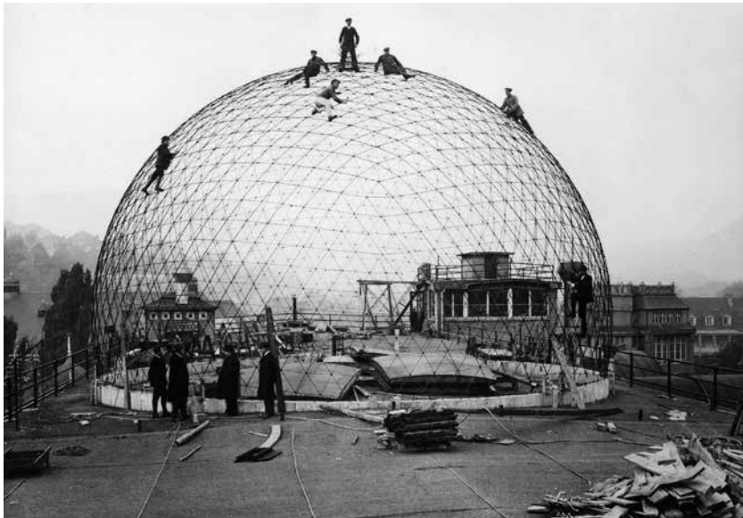
Figure 13.2 Construction of the Zeiss Planetarium in Jena, 1924
